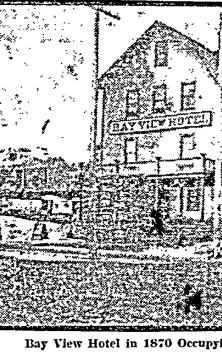
Bay View Hotel in 1870 Occupying the Site of the Palladio.
